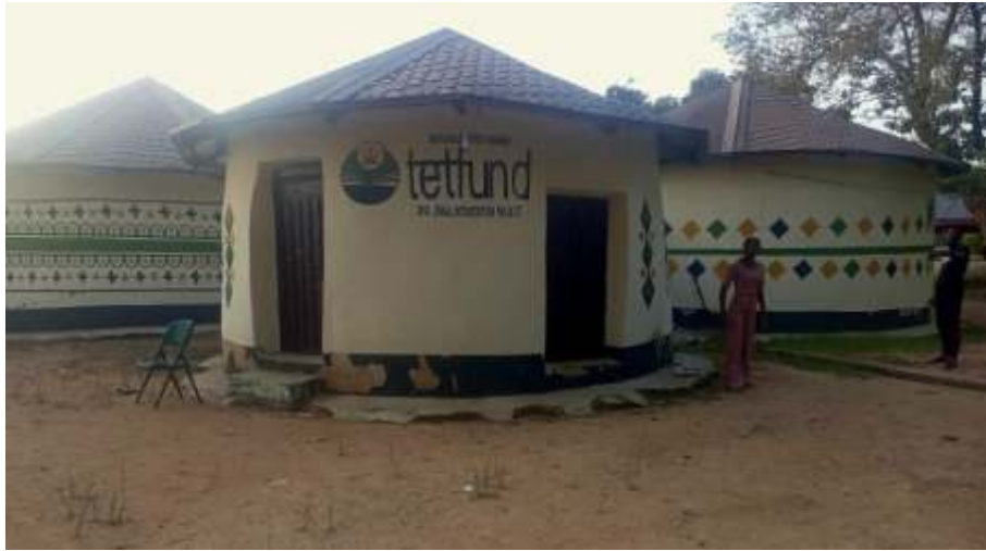
Fig. 4: The entrances into the renovated ABU Studio Theatre revealing its cyclical nature with roofs to simulate traditional grass patterns.
