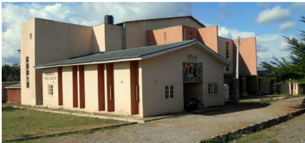
Fig. 6: The magnificent 1,500 capacity Theatre at FUOYE which has proscenium stage. This theatre stands as one of the biggest theatres in Nigerian Universities where Theatre Arts discipline is studied. Photo: The author – 16 June, 2023.
